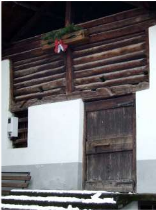
4. Tamponamento in block-bau
